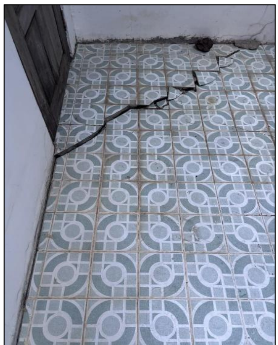
Figure 1.10 Settlement of Ground floor
