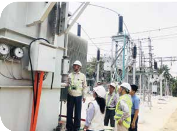
Dagon Seikkan Township, 66/11 KV, 20MVA Yuzana HGIS Sub-Station, Extension of 20 MVA Transformer (2021-2022)
