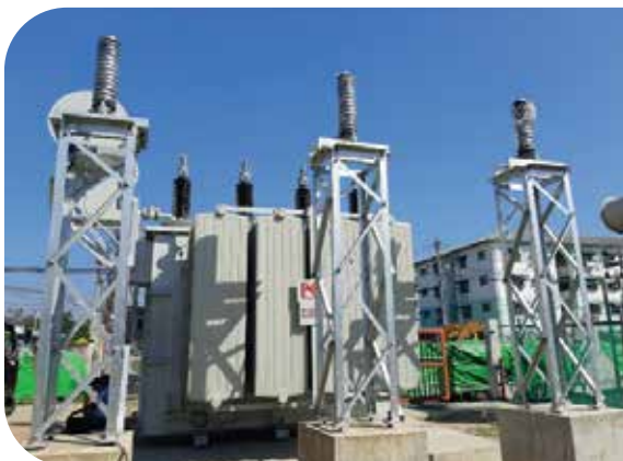
Dagon Seikkan Township, 66/11 KV, 20MVA Yuzana HGIS Sub-Station, Extension of 20 MVA Transformer (2020-2021)
