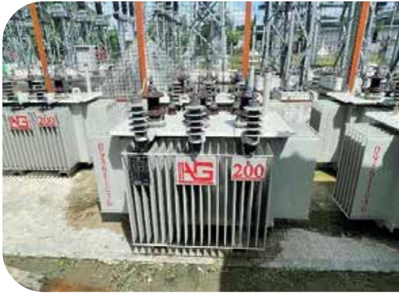
Dagon Seikkan Township, Yuzana Low Cost Housing Project, Lot-4, Installation of 11/0.4 KV, 200KVA Transformer-7 nos and Power Line (2020-2021)
